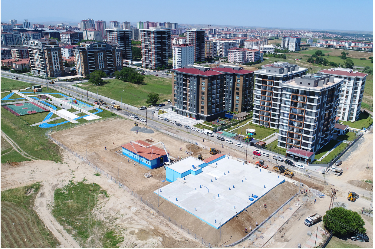
İçmesuyu Deposu ve Terfi Merkezi General View of Potable Water Cistern and Pumping Station
