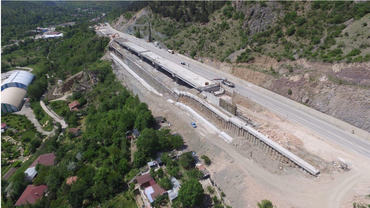
Köprü ve Kazık İmalatları Bridge and Bored Piles Construction
