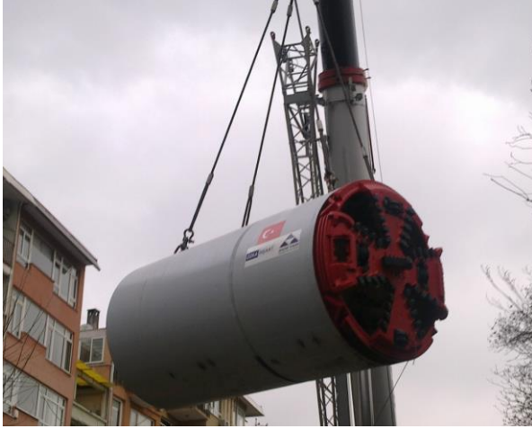
TBM Makinesi TBM Machine
